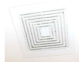
Keep exhaust fan clean
