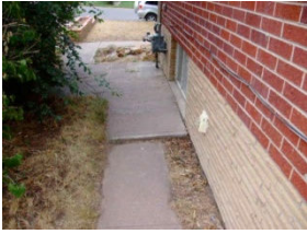
Concrete slopes to foundation
