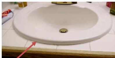
Caulk around sink
