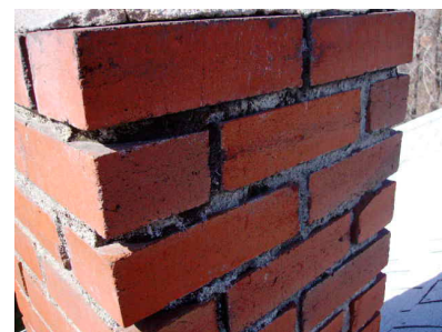
Deteriorated mortar
