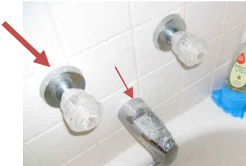
Caulk around spout and handles
